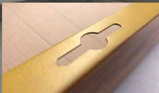
HIDDEN SHAPED LOCK FOR PANEL FIXATION
